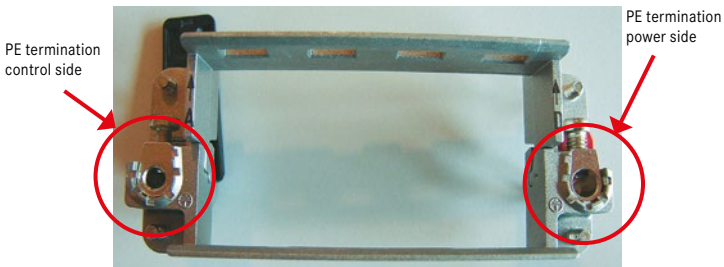
Figure II-3: Hinged frame - termination sides
